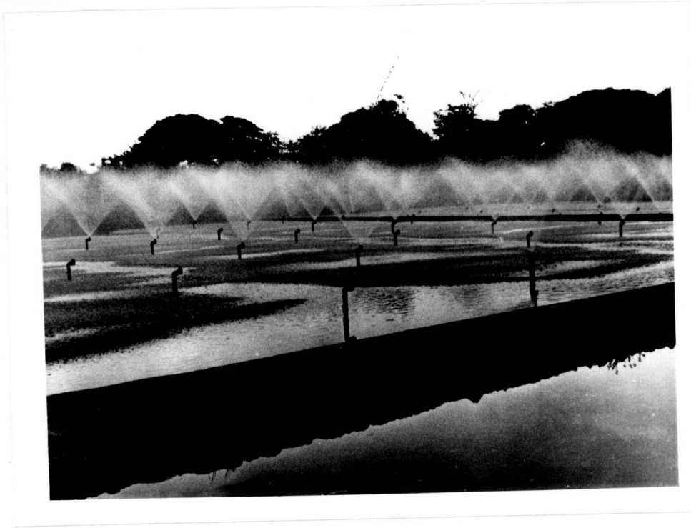
Plate 13 Treatment of Wastewater from Foremost Milk Factory through Sprinkular Aeration.
