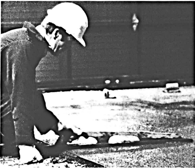
Fig. 26. Darbying brings the surface to the specified level.
