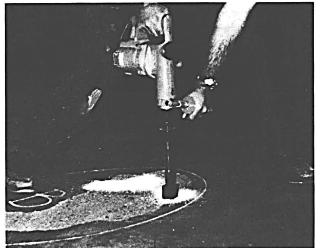
Fig. 34. Weak, defective concrete can be removed with a chipping hammer.
