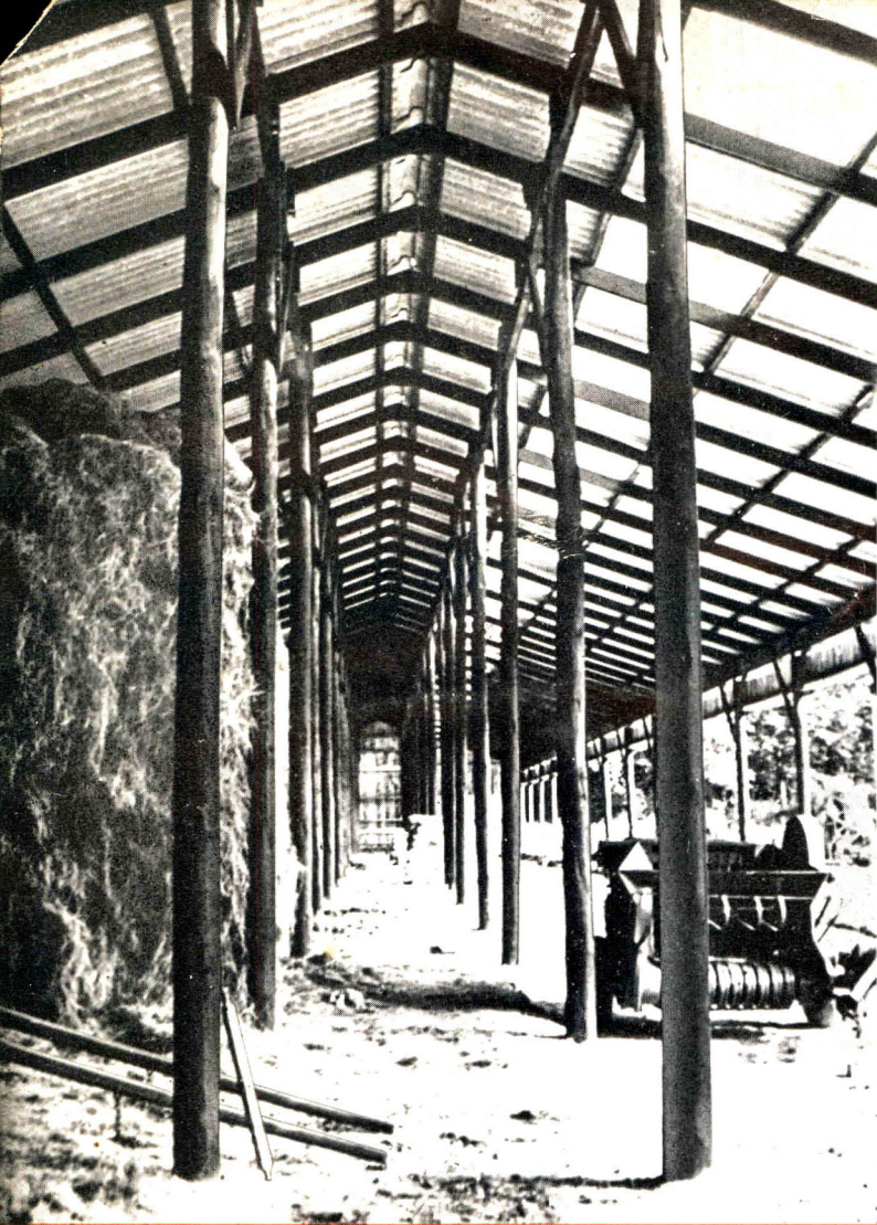
Pole type barn with pressure creosoted softwood poles as the main supporting timbers.
