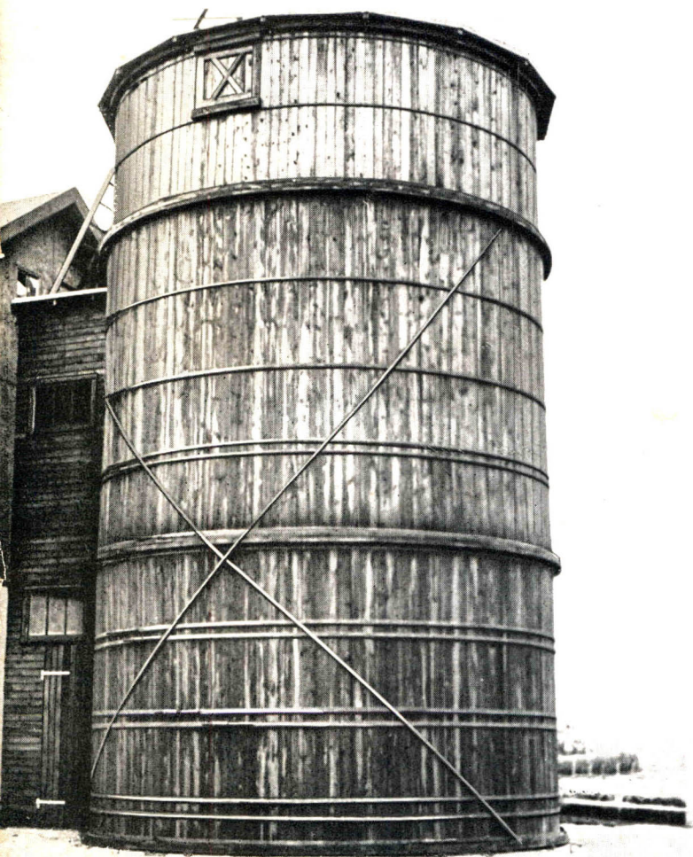
Silo constructed of pressure creosoted timber.
