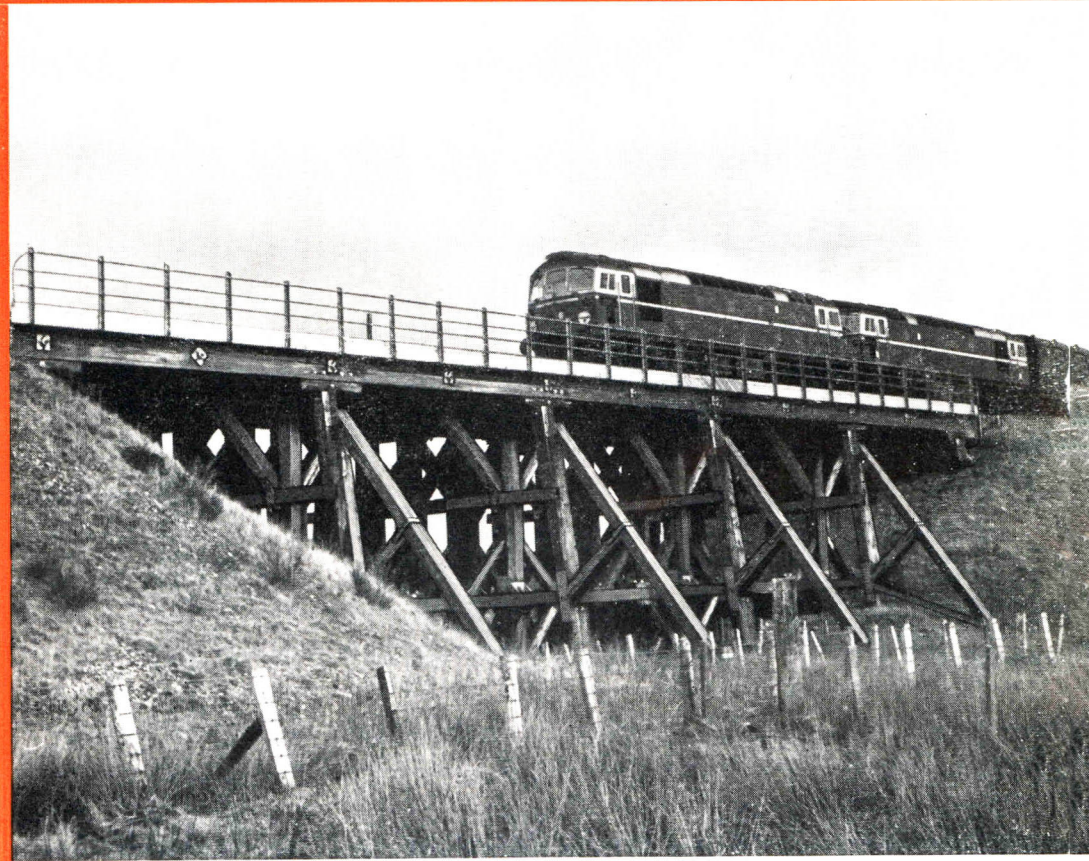
Creosoted wooden railway bridge constructed in 1894 and still in service on British Rail.
