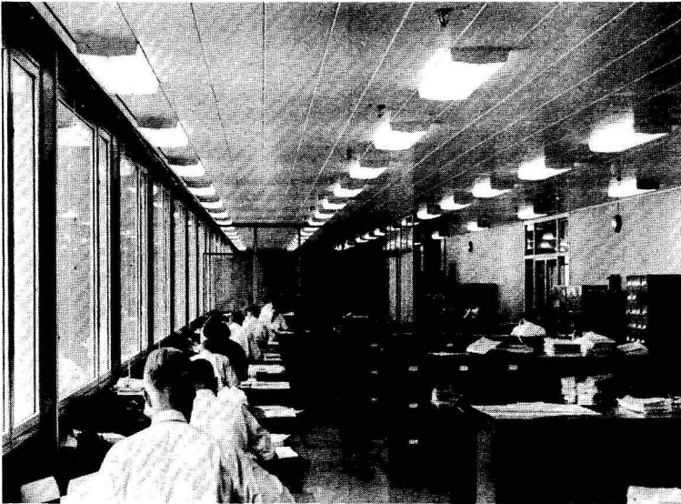
Fig. 25. - Since office workers normally sit side-on to the windows, fluorescent fittings should be placed parallel to the window wall, with the outermost row as close to it as possible
