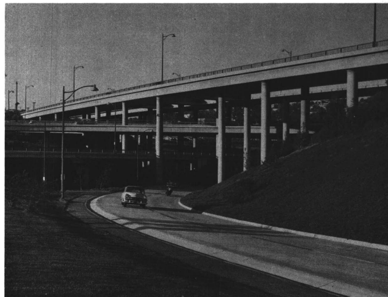
Fig. 10. Long spans and shallow superstructures are provided by box-girder construction in the top two levels of this multi-level grade separation in Los Angeles. Design: California State Department of Public Works, Division of Highways. Construction: James I. Barnes Construction Co., Santa Monica, Calif.
