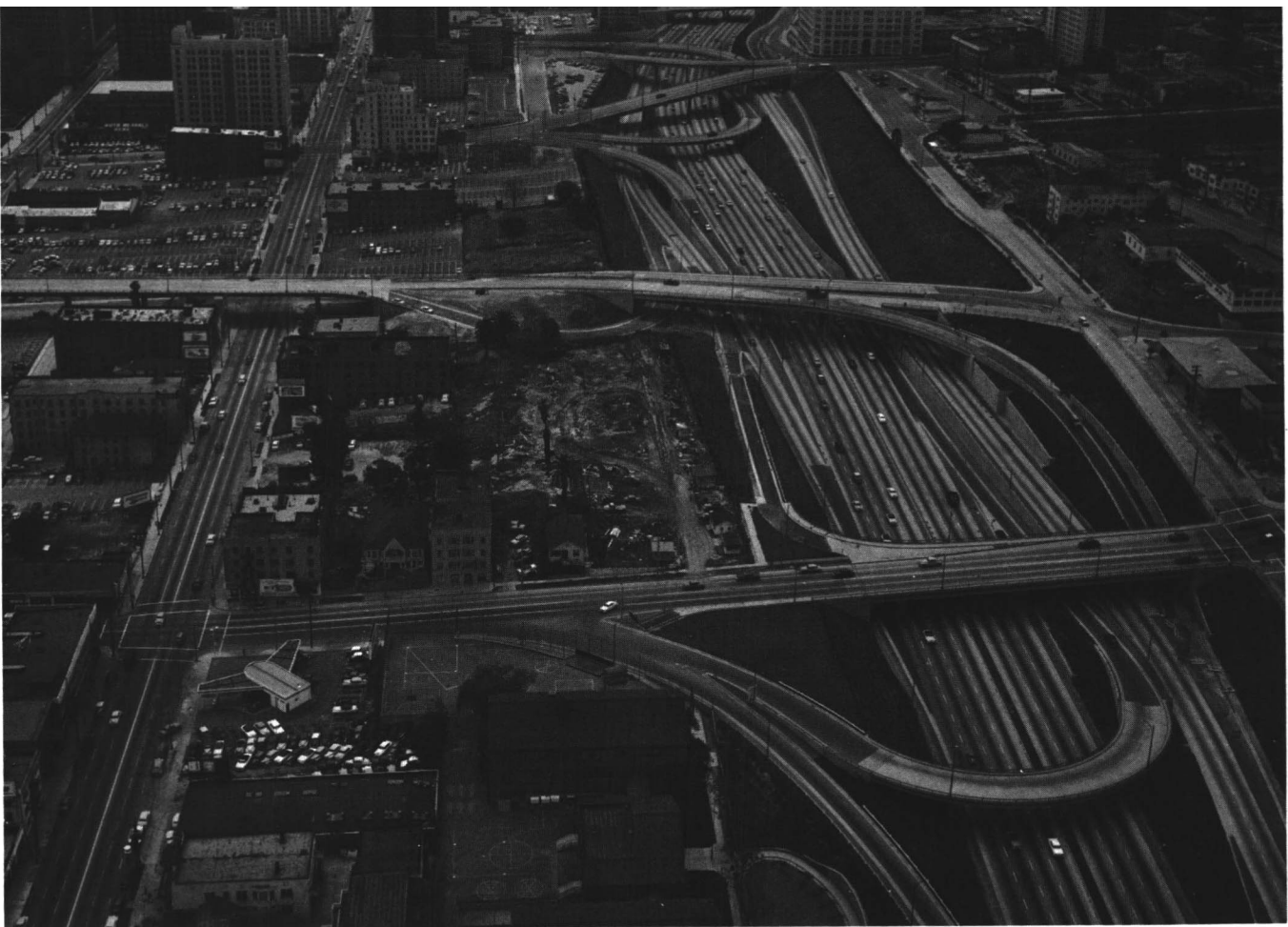
Fig. 3. Service roads for local traffic both flank and pass over the Los Angeles Harbor Freeway through busy industrial and residential areas. Interchange is by means of one-way ramps. Courtesy of California State Department of Public Works, Division of Highways.
