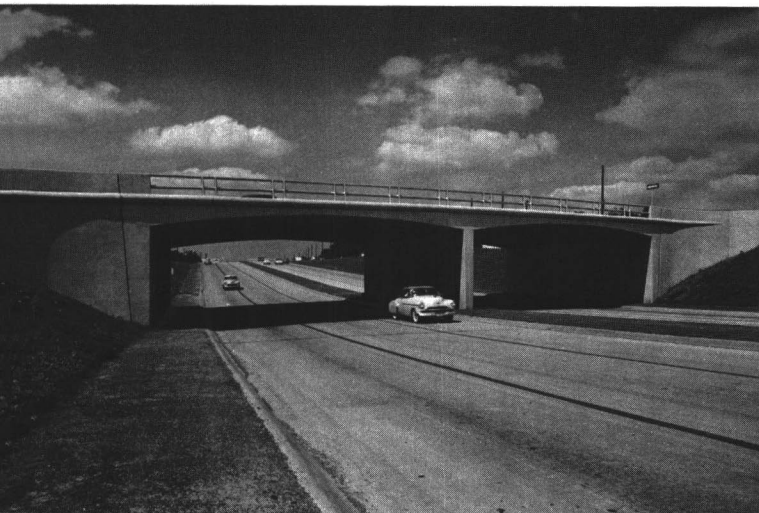
Fig. 15. Maximum driving safety is provided by carrying the full roadway width, including shoulders, under structures on the Dallas Central Expressway. Design: Texas State Highway Department. Construction: Austin Bridge Co., Dallas, Texas.
