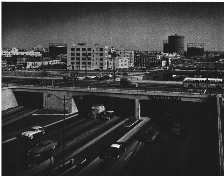
Fig. 8. Vertical clearance and right-of-way limitations were easily satisfied by the use of rigid-frame box-girder construction for these bridges in Los Angeles, Calif. Design: City of Los Angeles. Construction: Guy F. Atkinson Co., San Francisco, Calif.
