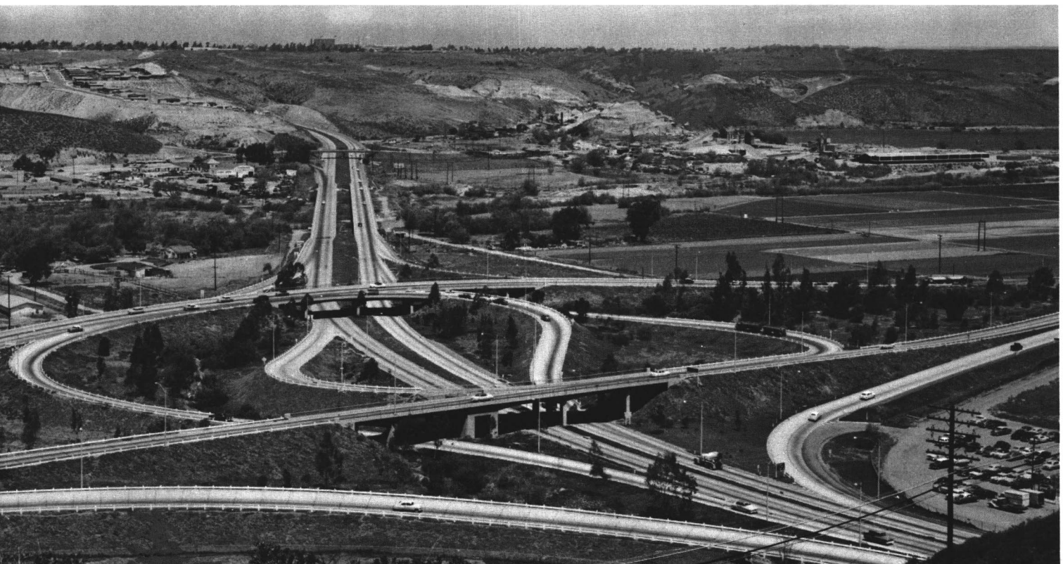
Fig. 2. This directional interchange at the intersection of U.S. 80 and the Cabrillo Freeway, San Diego, Calif., allows vehicles to change direction with little reduction in speed and without obstruction to through traffic.
