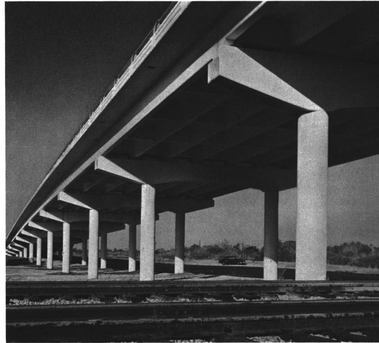
Fig. 18. Site-casting the 192 posttensioned 60-ft. girders needed for the Wisner Blvd. Overpass, New Orleans, La., reduced handling to a minimum. Precast diaphragms were used between the beams, which were set 6 ft. 8 in. apart. Design: George A. Heft & Co. Construction: Keller Construction Corp. Both are of New Orleans.
