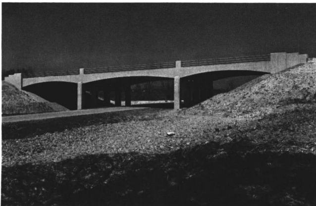
Fig. 5. Maximum visibility is provided by this bridge in St. Clair County, Ill., which has open piers and open end spans with spill-through abutments. Design: Illinois Division of Highways. Construction: Maurice Hoeffken Co., Belleville, Ill.
