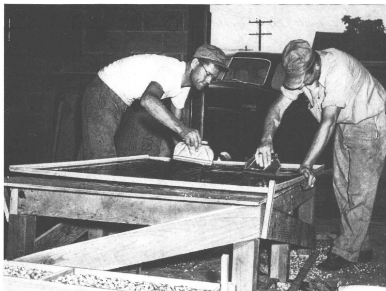
5 A special adhesive is spread to a uniform depth on a liner panel with toothed trowels.
