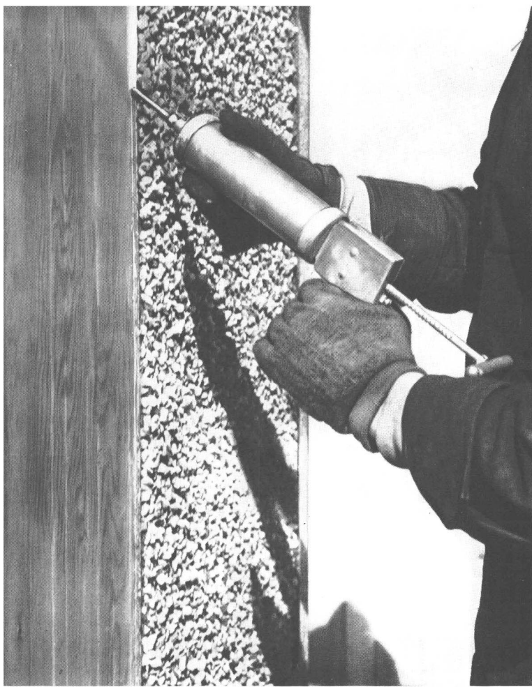
13 Caulking compound is used to seal joints between panels; an excess amount should be avoided.
