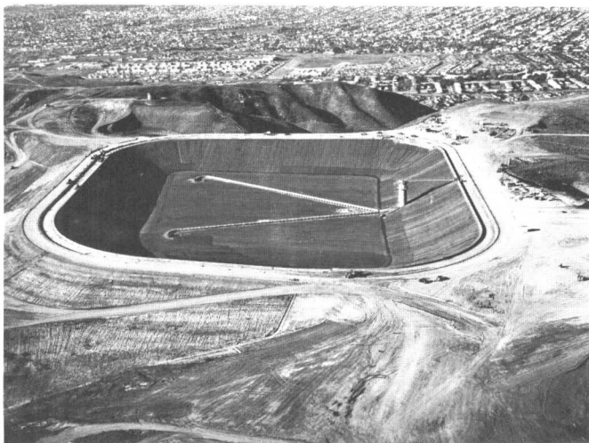
Figure II-12—Asphalt Lined Baldwin Hills Reservoir, Los Angeles
