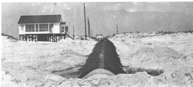
D. Completed Groin
