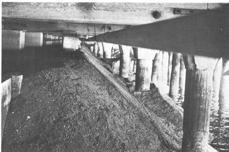
Figure IV-5—Seawall, Los Angeles Harbor (Photographed in 1960)
