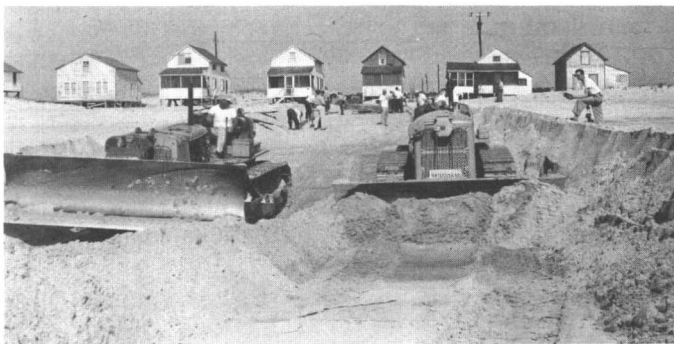
A. Dozers Preparing Excavation
