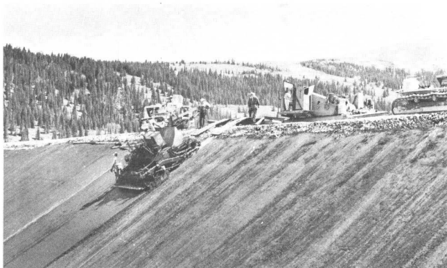
Figure V-7—Montgomery Dam—Tractor Drawn Turntable and Paver at Top of Dam
