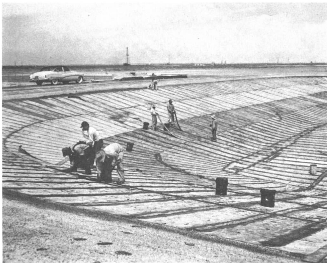
Figure II-33—Prefabricated Asphalt Panel Lining under Construction
