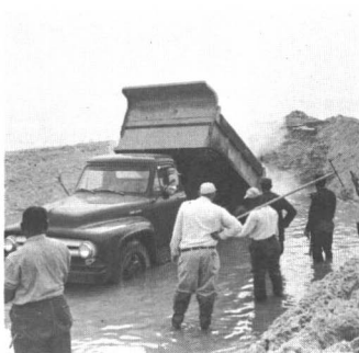
B. Truck Dumping First Load of Hot-Mix at Seaward End
