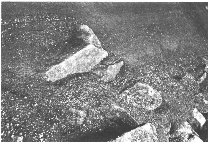
Figure IV-4—Seawall, Los Angeles Harbor (Showing texture of asphalt and embedment of stone)
