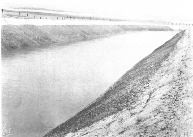
Figure II-29—Asphalt Macadam Cover Over Asphalt Membrane
