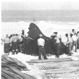
C. Workers Shaping Upper Structure of Groin
