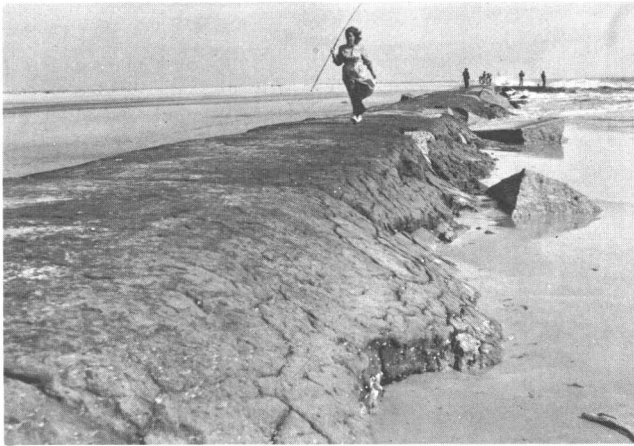
Figure IV-3—Galveston Jetty After Fifteen Years' Service
