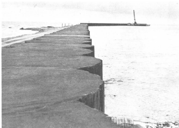
Figure IV-11—Asphalt Capped Cellular Breakwater, Port Austin, Mich.
