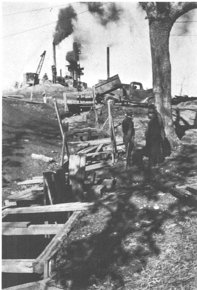
V-11—View of Top of Trench, Claytor Dam
