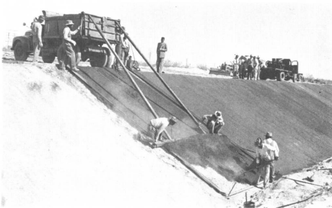
A. Improvised Strike-Off Screed
