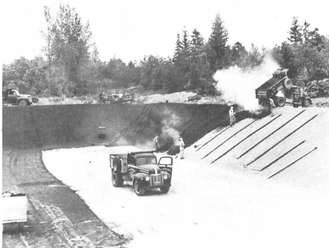
Figure II-10—Paving Slope by Improved Methods
