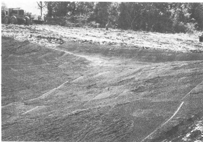
Figure III-6—Detail for Surface Drainage, Upper Bank Paving (Note texture of uncompacted sand asphalt revetment)
