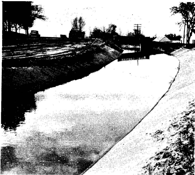
Figure II-5—Asphalt Concrete Lined Canal
