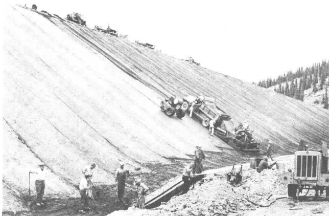
Figure V-6—Montgomery Dam, Colorado—Paving and Compacting Operations (Note cut-off wall)
