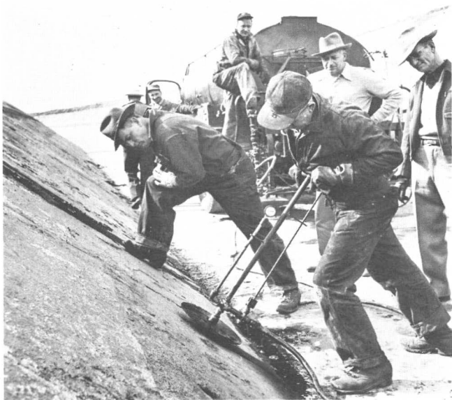
Figure II-27—Undersealing Portland Cement Canal Lining with Asphalt
