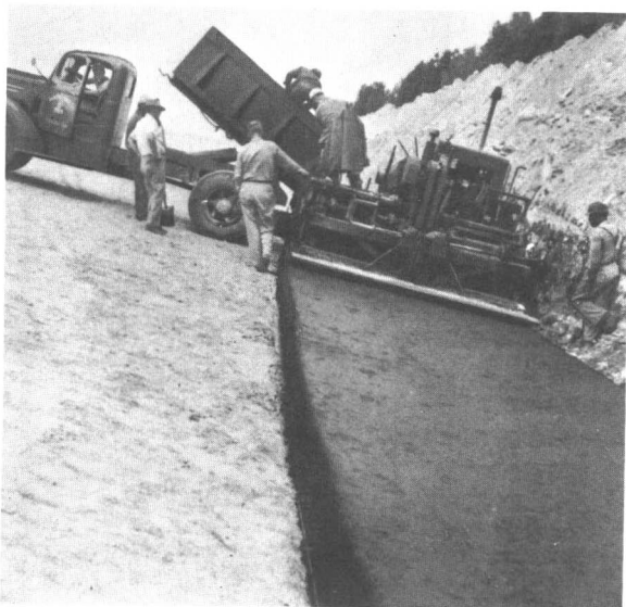
Figure III-8—Paving Machine at Toe of Slope, Lake Okeechobee
