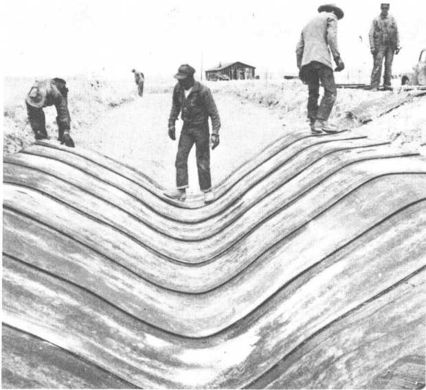
Figure II-34—Lining Ditch with Prefabricated Asphalt Panels
