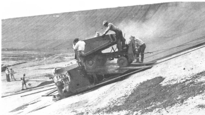
Figure II-9—Special Slope Paver and Hopper Car
