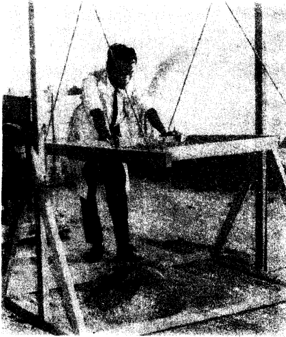
Figure 3. Screening pulverized soil.
