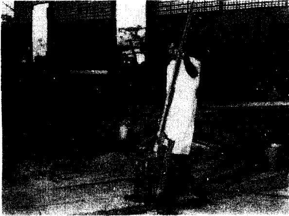
Figure 7. Swinging moulder lever to vertical position to allow compaction to begin.
