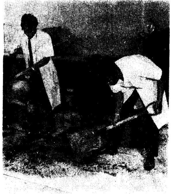
Figure 4. Mixing cement and soil.
